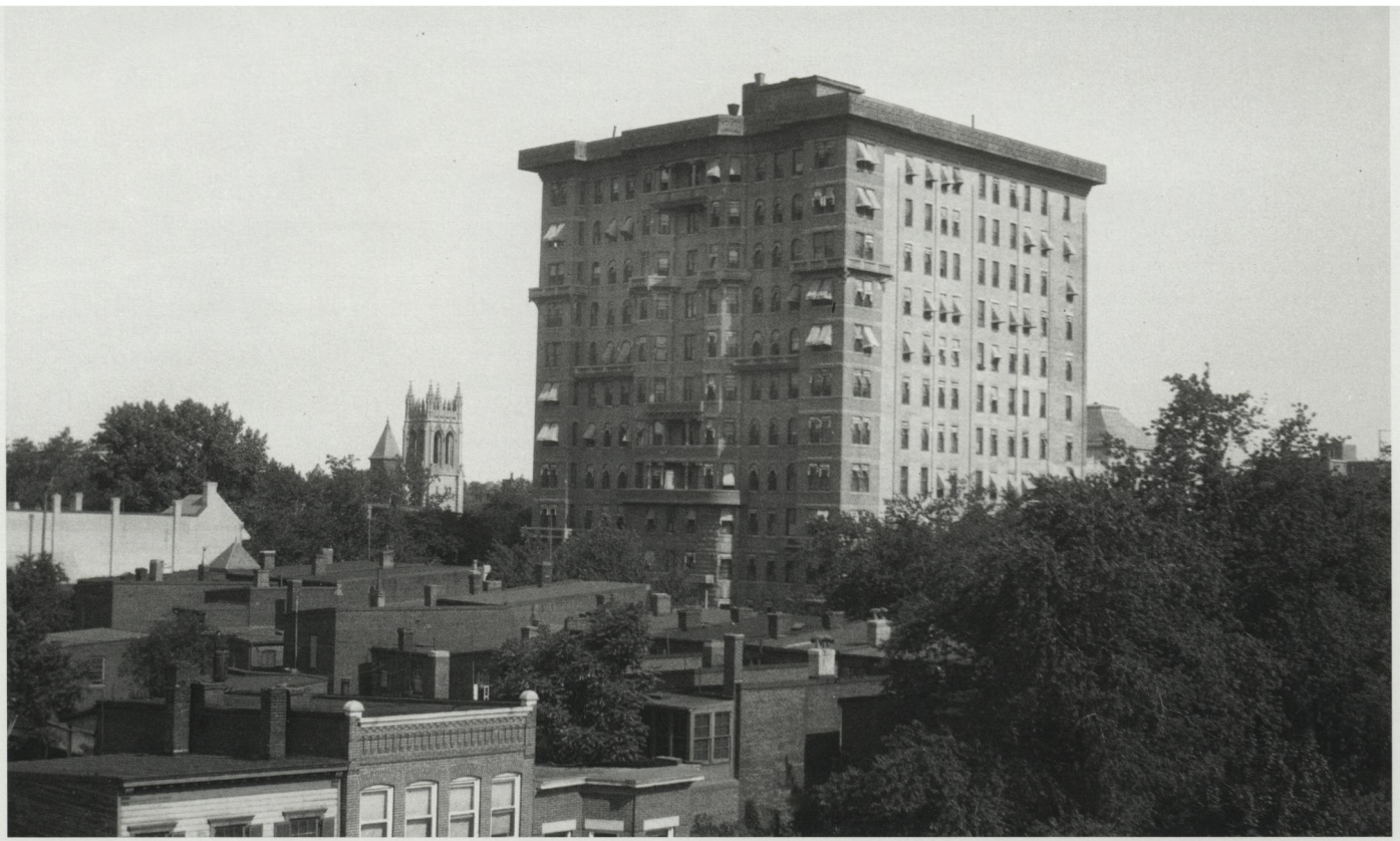
The Cairo Hotel looms over its neighbors in this view from the 1960s. Historical Society of Washington, D.C.
